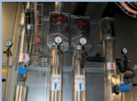
SUPI offers the complex inspection and expertise
